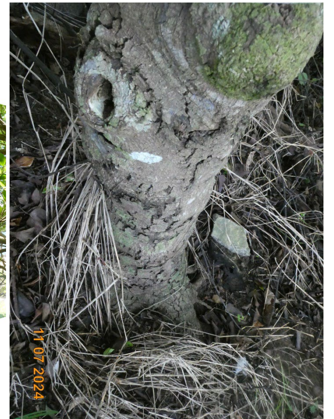
Photo No. 16 | T80 (Fell)
