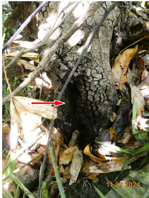
Photo No. 5 | T71 (Fell)
